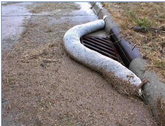
Some methods are not allowed. These methods include using filter fabric installed under the inlet grates and the use of straw bales. Non-porous materials are to be avoided.
