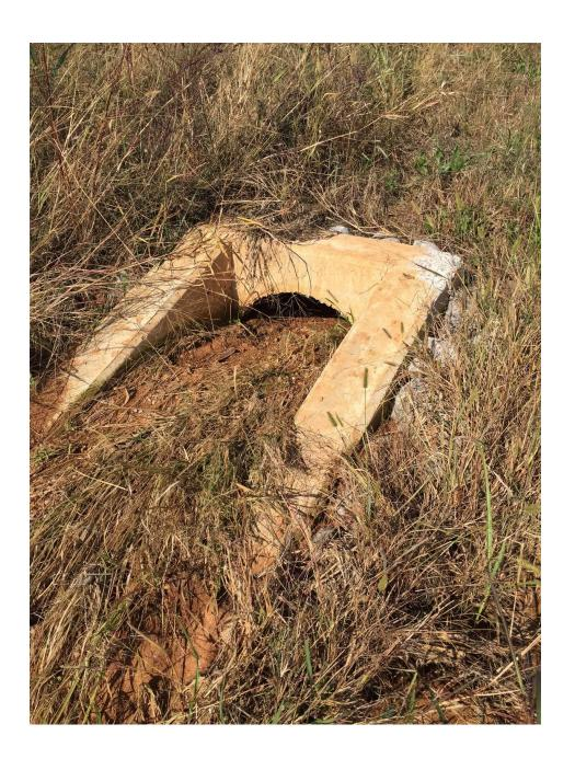
Poorly vegetated swales can lead to erosion damage and property value loss. Water can be polluted by sediment released in the erosion process
