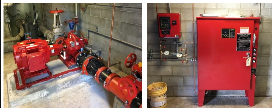
New fire pump controller, jockey pump, and control panel 12/16
