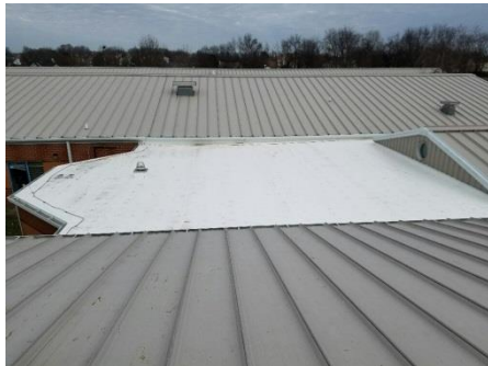
Hazelwood Sarnafil Roof and Gutters 12/16
