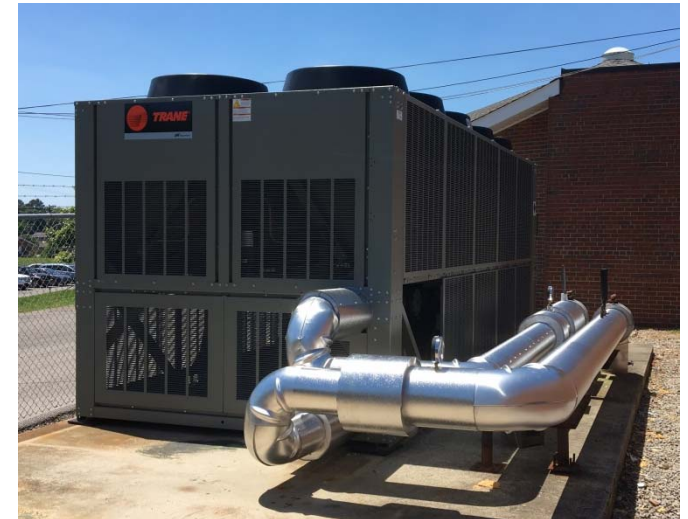
Moore Replacement Chiller Installed 6/17
