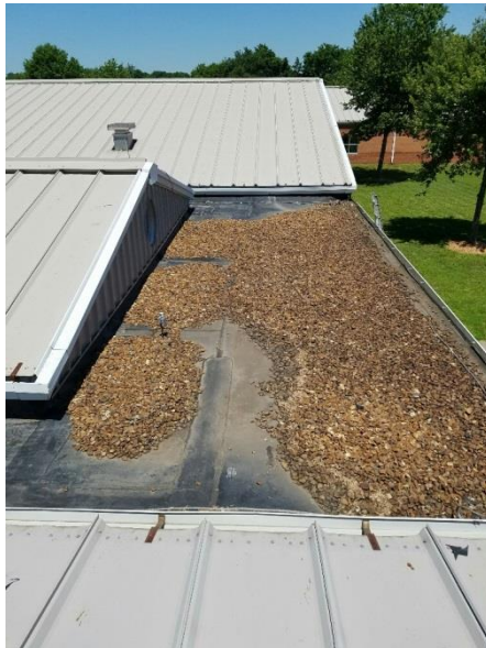
Current condition of Hazelwood Ballasted EPDM Roof 6/16
