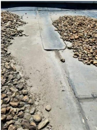
Current condition of Hazelwood Ballasted EPDM Roof 6/16
