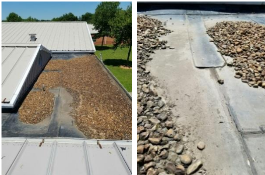
Current condition of Hazelwood Ballasted EPDM Roof 9/16
