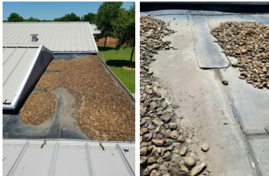
Current condition of Hazelwood Ballasted EPDM Roof 9/16
