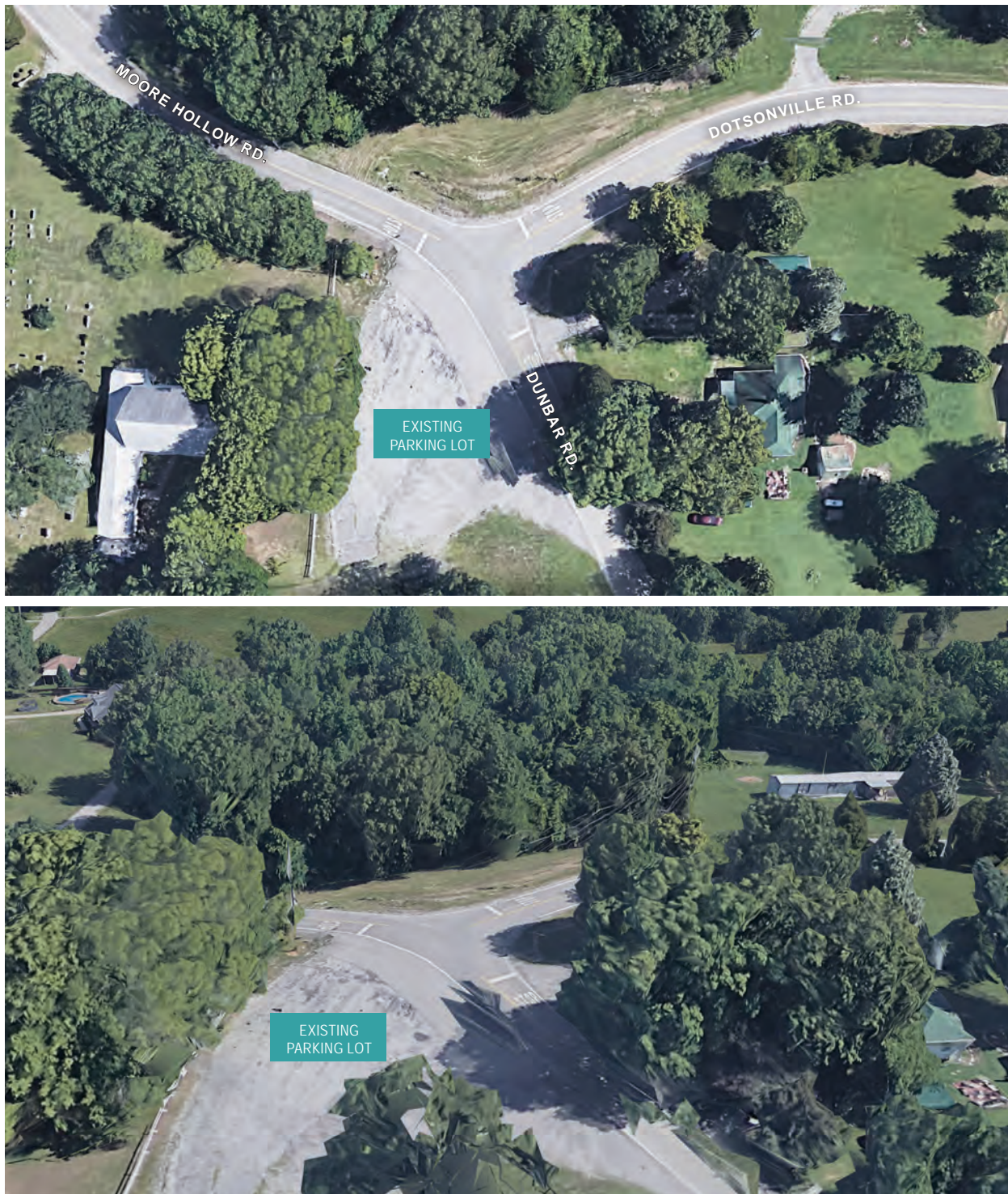
Figure 9a: Dotsonville Road existing conditions, plan view and axonometric view above. Refer to Figure 8 (pg. 11) for location on HIN map (L13).
