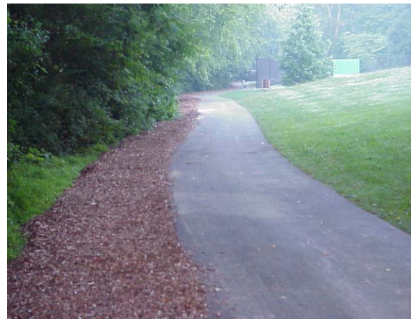
Figure 1.15: Temporary access road widening
