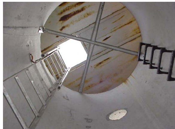
Figure 1.13: Ladder and steps in riser.
