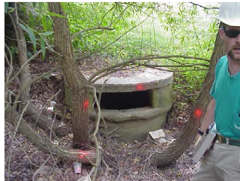
Figure 2.2: Marking trees to be removed.
