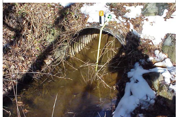
Figure M6.3: Forced access location.
