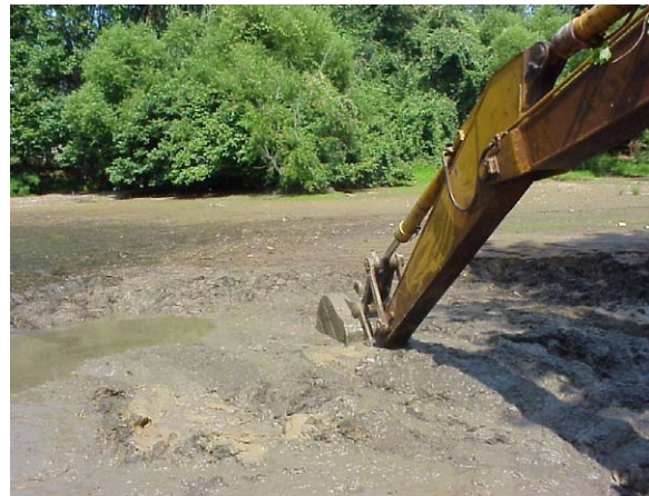
Figure M5.4: Mechanical dredging with backhoe.
