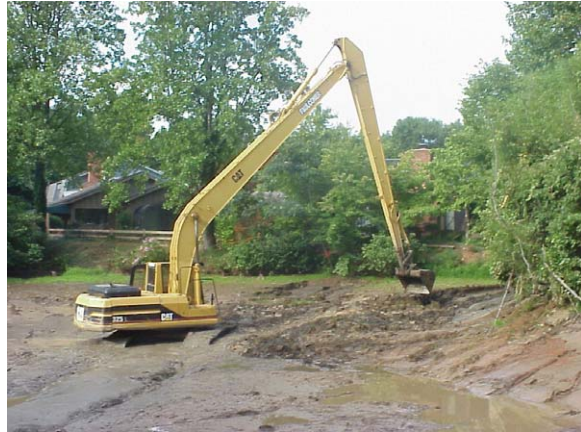
Figure 1.11: Muck removal and slope dressing by long reach backhoe
