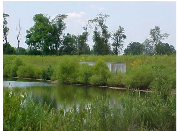
Figure 1.9: Excessive vegetative growth obscures riser
