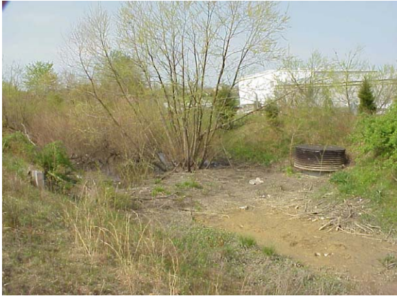
Figure 1.10: Sediment accumulation in a dry pond
