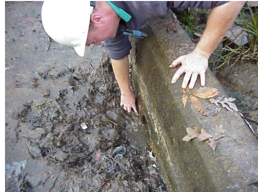
Figure M2.3: After clog is removed.
