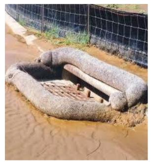
downstream inlet. For example, silt fence that has not been properly trenched around the inlet can result in flows under the silt fence and directly into the inlet.
